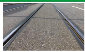
Corabit S is a polymer-modified, bituminous compound in accordance with TL/TP Fug-StB 15 and is used for joints between rails and adjacent coverings such as paving, asphalt or concrete without special chemical
